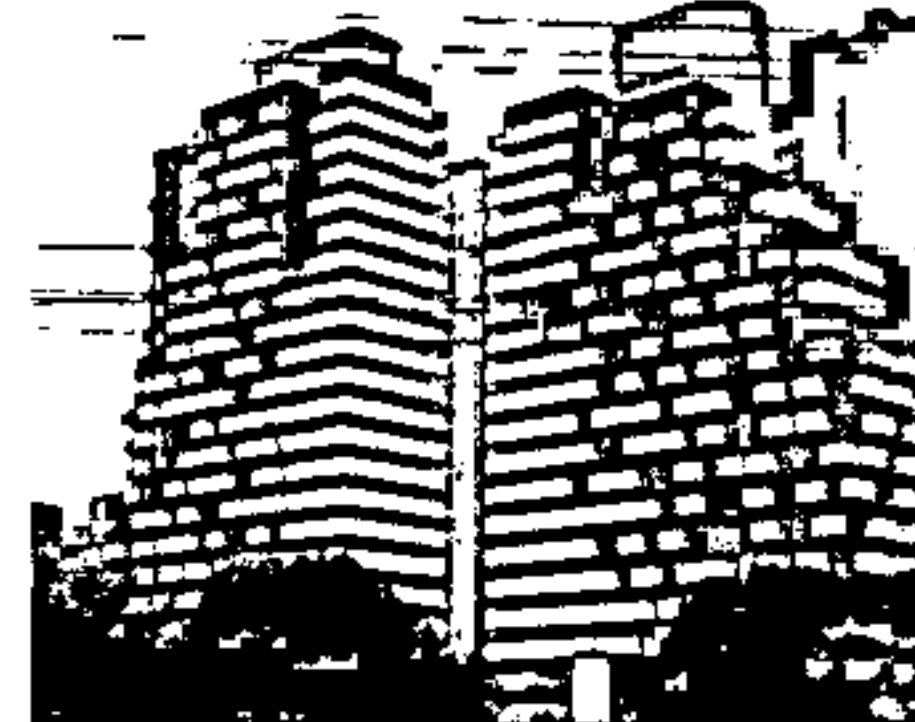
Top Towers Offices
