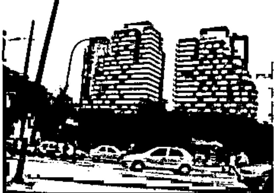
Top Towers Offices
